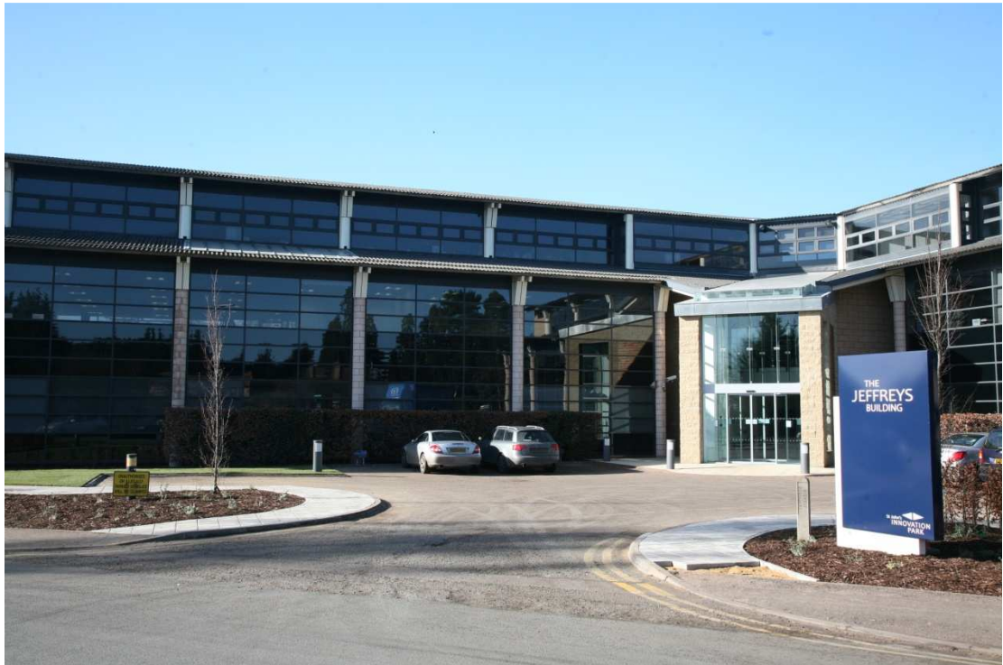
The Jeffreys Building, St John's Innovation Park
