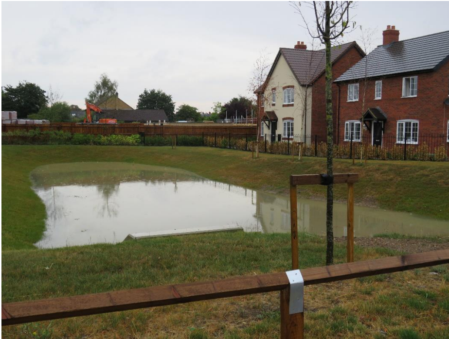
Figure 6.11: Drainage basin created as part of new development along Bannold Road
