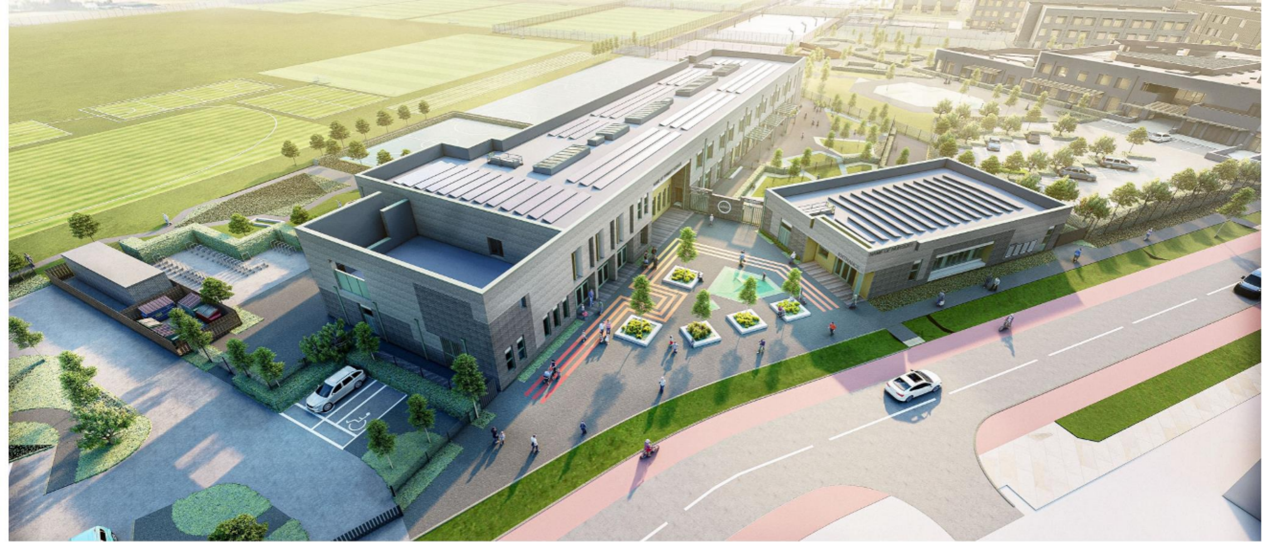
AERIAL VIEW LOOKING SOUTH
