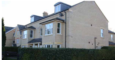
Blonde brick façade in contemporary dwelling
