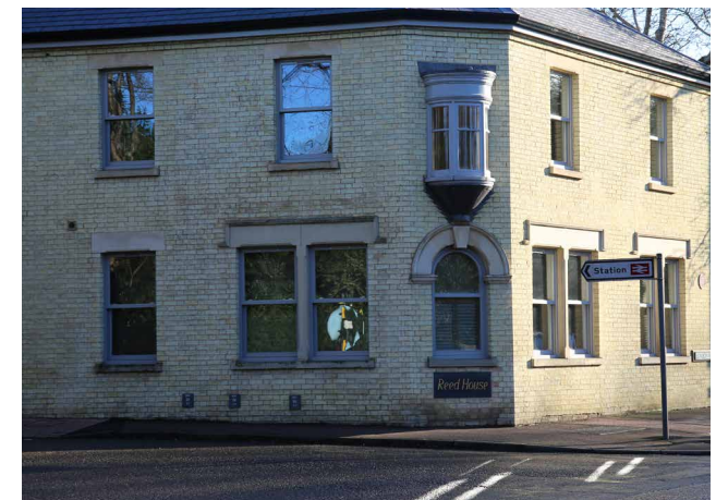
Figure 03: Office at junction of Station Road and London Road.
