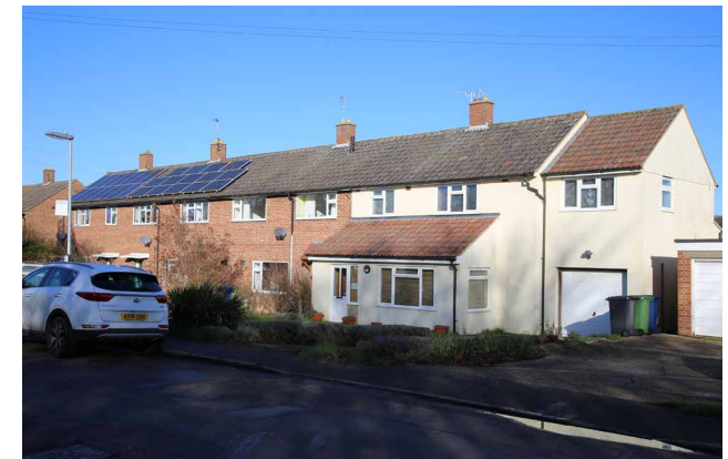
Figure 70: Example of an unsympathetic front extension which substantially changes the building line and interrupts the unified nature of the existing terrace.
