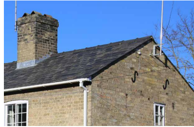
Slate tiles on gabled roof
