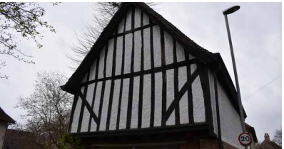
Timber frame gable wall with rough cast render
