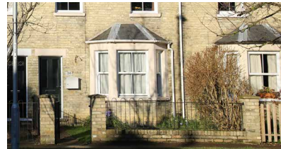
Bay vertical sash windows
