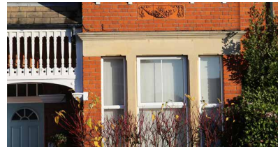
Redbrick façade with limestone lintels
