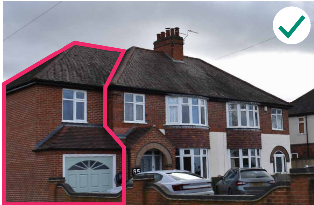
Figure 65: Outside example of a side extension.
