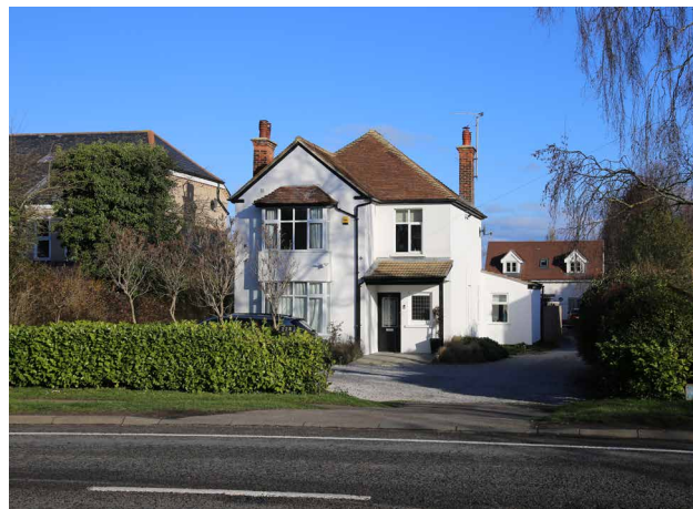
Figure 28: Example of a row of brown brick semi-detached dwellings (top).
