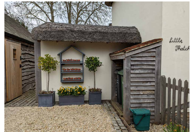
Figure 95: Outside example where the bins are stored under the shed, whilst the side wall is decorated with flowers and plants to improve the environment.
