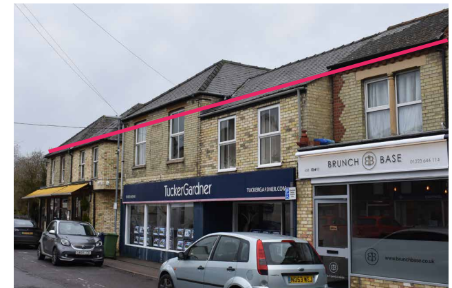
Figure 63: Example of shallow roofs with standard edge on Woollards Lane.
