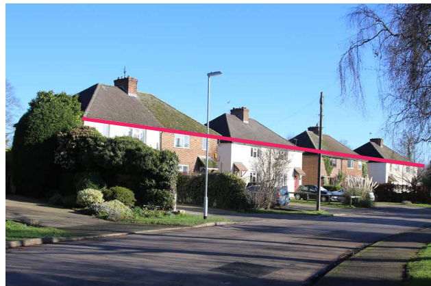
Figure 62: Example of typical hipped roofline in Stapleford.
