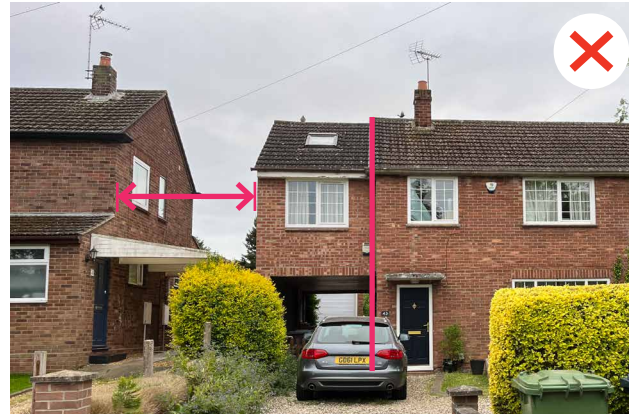
Figure 66: Local example of an side extension.
