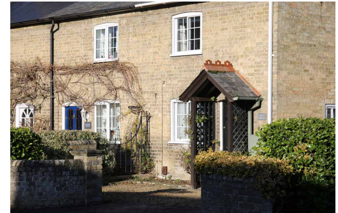
Figure 69: Local example of a porch which is in keeping with the simple form of the existing dwelling and features a sympathetic material palette.
