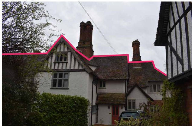
Figure 61: Example of an asymmetrical and complex roofline in Great Shelford.
