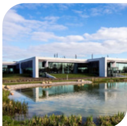
East Anglia regional winner for best non-residential new build, Project Birchwood, Melbourn Science Park. Project Team: SDC Builders, Sheppard Robson, TTP, 3C Shared Services Building Control
